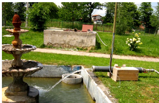
Opitno crpljenje bunara termomineralne vode lječilišta "Gata" Bihać / Pumping test of termomineral water well at the healing resort "Gata"
