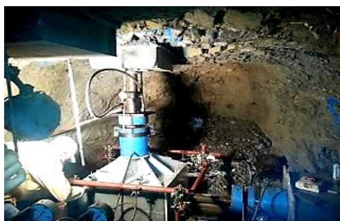
"In situ" geotehnička ispitivanja za objekat hidrocentrale "Vranduk" na rijeci Bosni / "In situ" geotechnical testing for hydroelectric power plant on river "Bosna"
