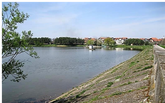
Tehnička osmatranja brana "Vidara" i "Hazna" u Gradačcu Technical monitoring of dams "Vidara" and "Hazna" in Gradačac
